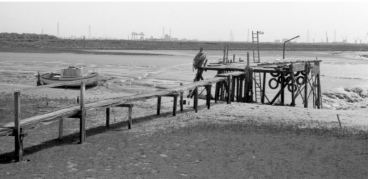
Jetty, Greatham Creek c.1972.
