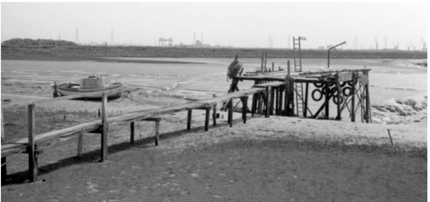
Jetty, Greatham Creek c.1972.
