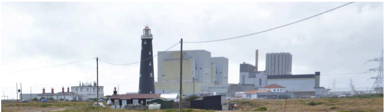
Dungeness nuclear power station.
