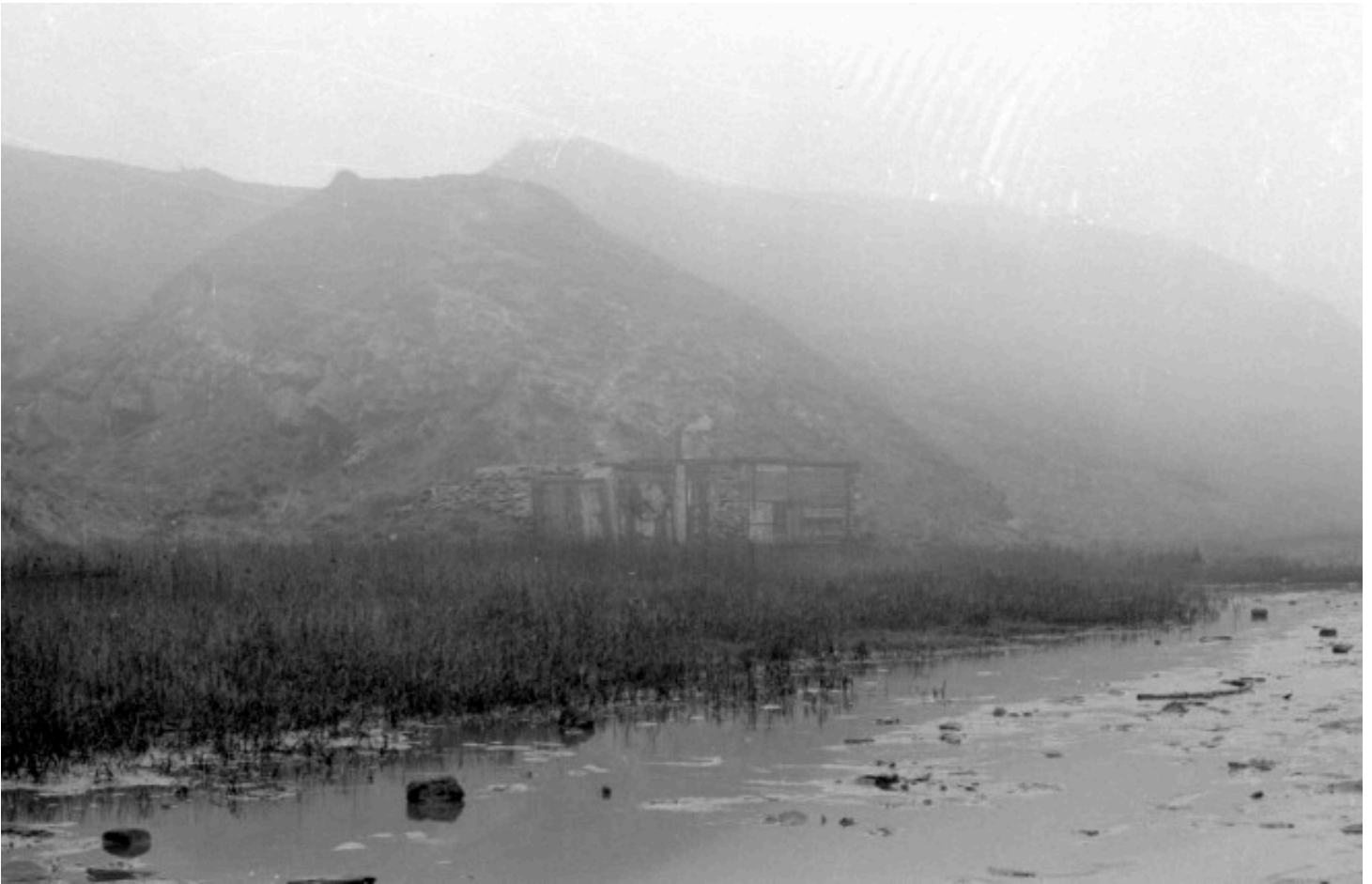
Timber hut (since destroyed). Blackhall Rocks 1973.
